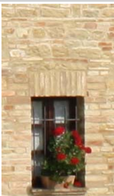
Lines of tiles kept the stone straight, and bars at the windows kept the animals safe.
