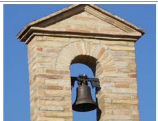
The original bell tower was rebuilt during the restoration, and a new bell commissioned.
